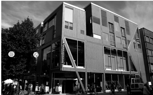
Figure 8: The new building which was constructed on the burn-out ruins. Photo: DK.
