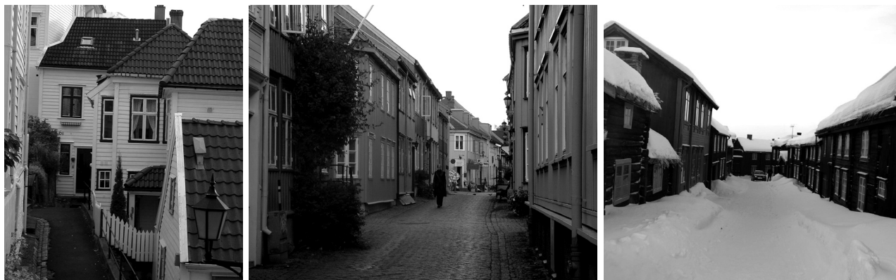
Figure 1: The wooden architecture reflects a more than thousand years old building tradition. From Bergen, Trondheim and Røros. Photo: DK
